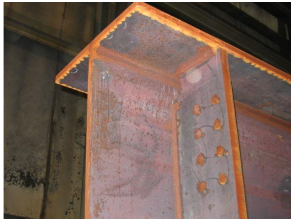
Figure 16 Photo showing a girder before blast cleaning
