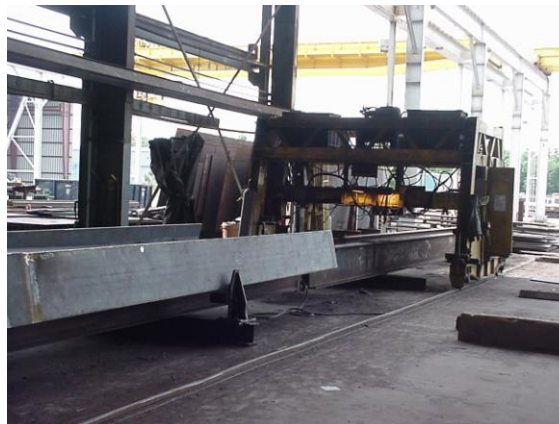
Figure 9 Photo showing the building of girders with their webs horizontal
