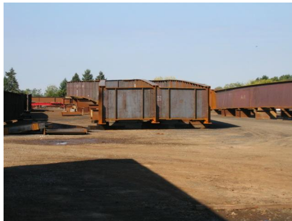
Figure 15 Photo showing the unit assembly of a structure
