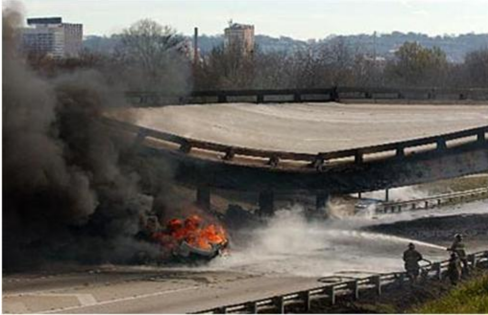
Figure 6 Fuel truck crash causes severe fire under the I-65 South over I-65 North overpass in Birmingham, Alabama, January 2002.
