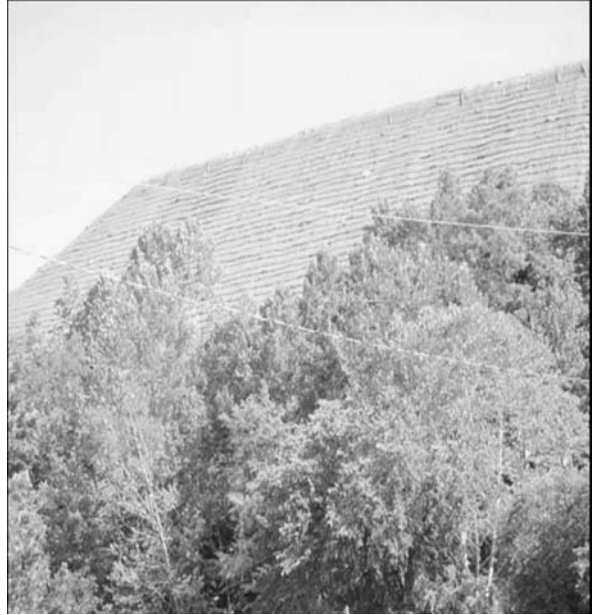
b) Slope face during construction.
