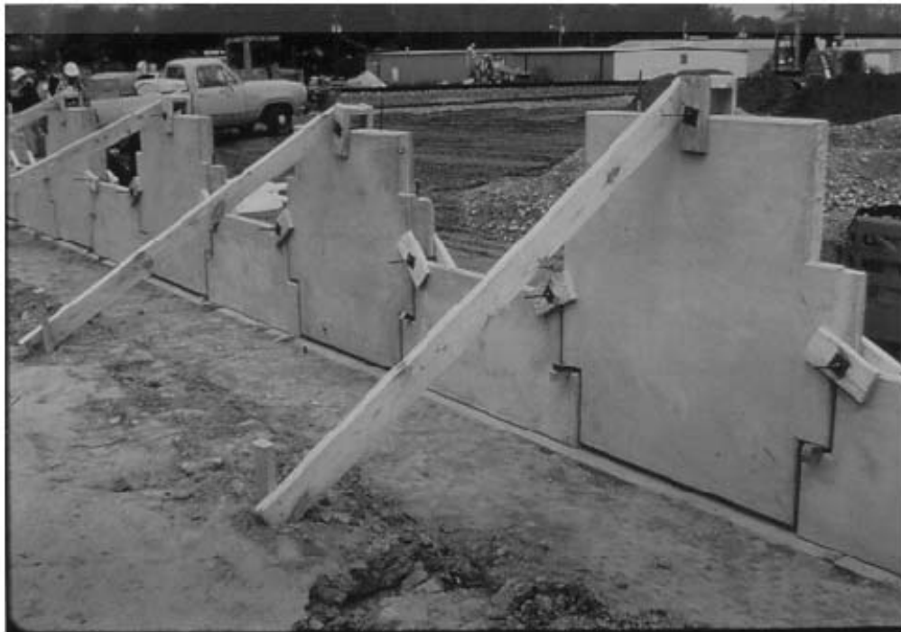
Figure 11-6. Setting first row of precast facing elements.
