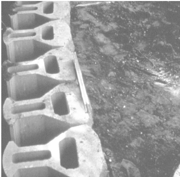
Figure 11-4. Checking facing element batter and alignment.
