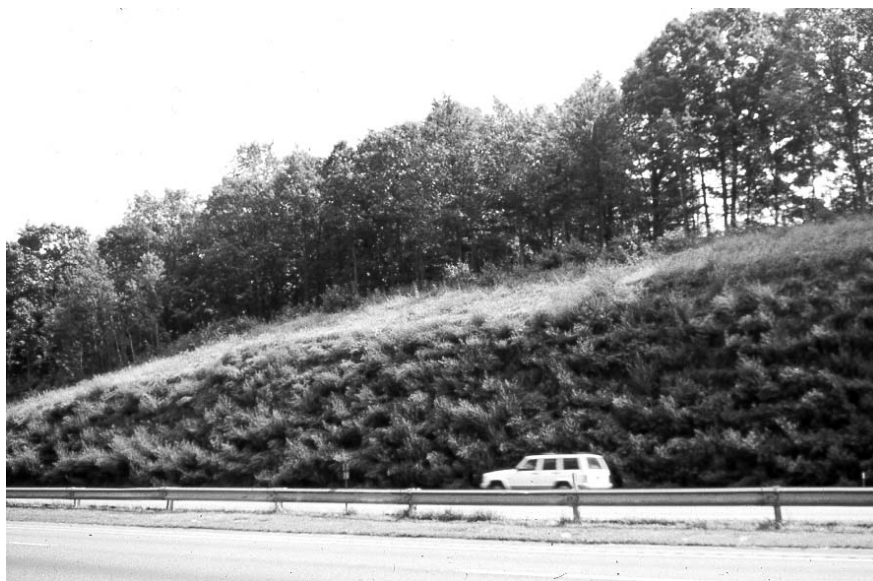
Figure 8-11. Massachusetts Turnpike during construction, immediately after construction and the after the second growing season.
