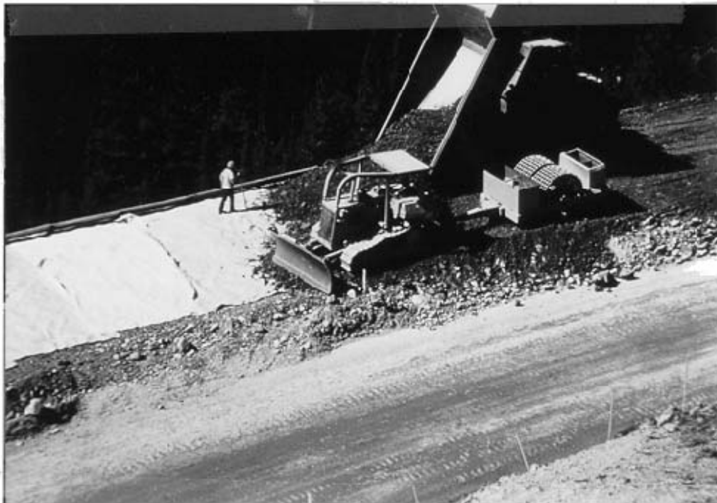
Figure 11-7. Placement of reinforced fill.
