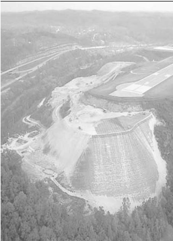
c) Aerial photo of slope during construction, approximately 80% complete.
