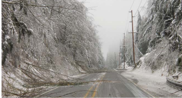
Photo courtesy of the Washington State DOT.
