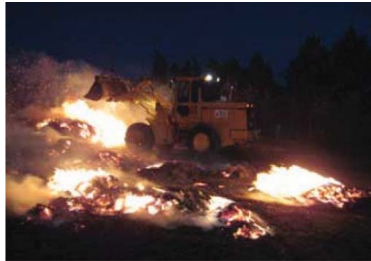
Photo courtesy of the Texas DOT.
