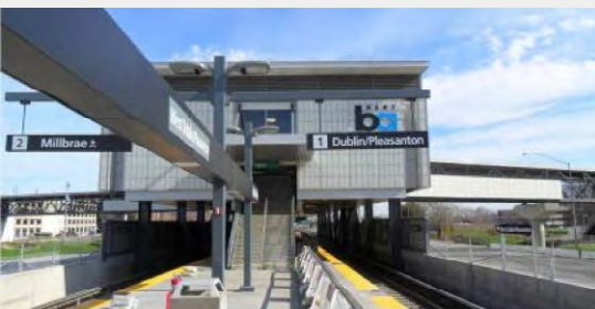
West Dublin/Pleasanton Station.
