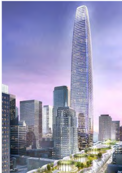
The Transbay Transit Center in San Francisco, CA.
