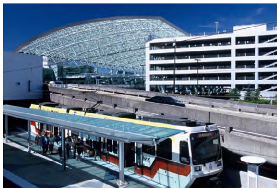
West Dublin/Pleasanton Station.
