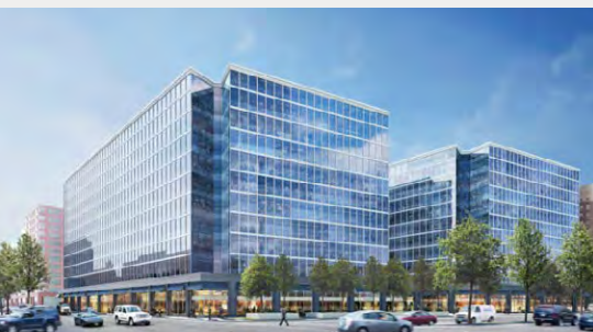
West Dublin/Pleasanton Station, Dublin, CA.
