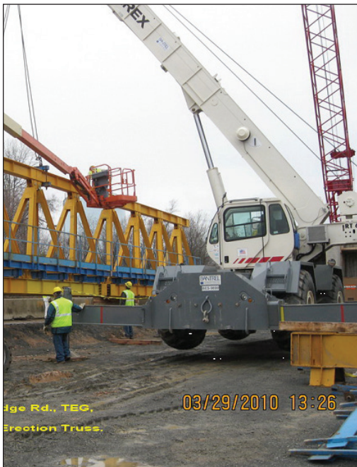
Dulles Corridor Metrorail Project construction, Northern Virginia
