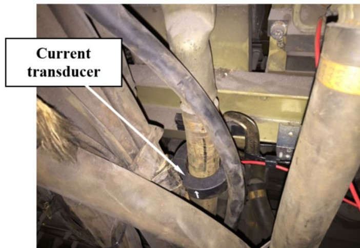
Figure 2-7. Current transducer installed around traction motor lead, GP-30 locomotives
