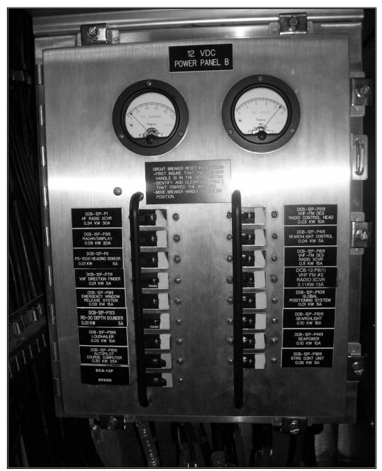
Figure 3-10 12 VDC Power Panel
