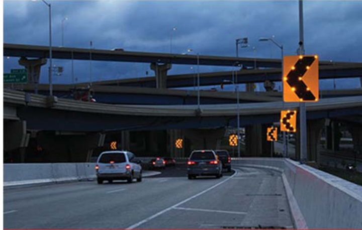
Figure 1. Photo. Sequential dynamic curve warning system.
