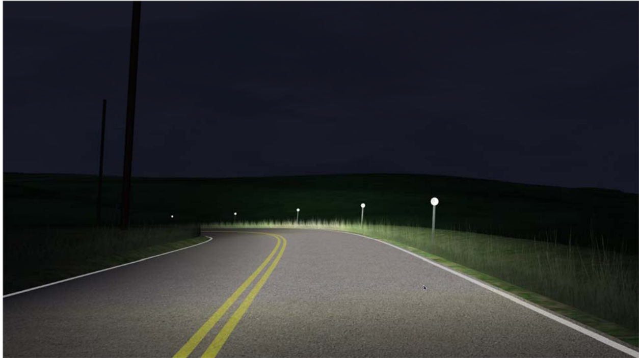
Figure 3. Photo. Example treatment-flashing in unison.
