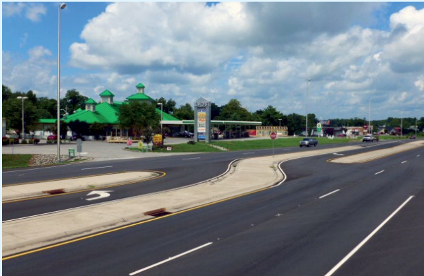
Restricting the direct crossing movement reduces the number of conflict points and severity of crashes.
