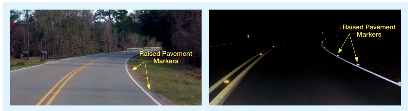
Example of 20 feet RPM spacing for a curve.
