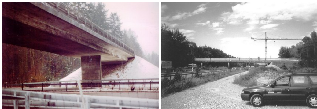
Figure 4.1: Views of the Z24 bridge
