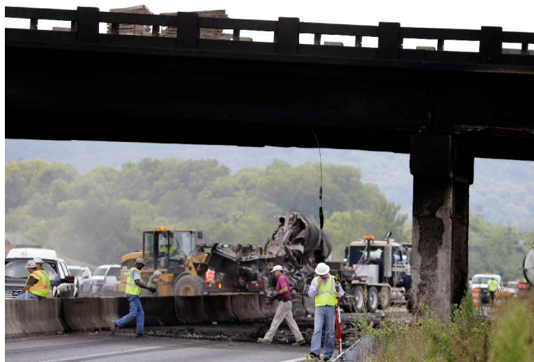
Figure 1.1 I-65 vehicle collision and explosion [1]
