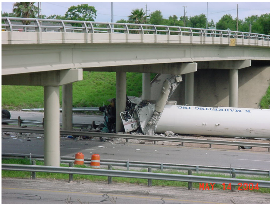
Figure 2.3 I-37 pier collision (6)
