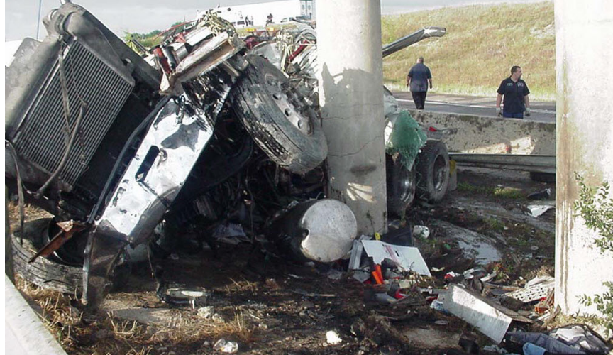
(a) Truck collision with RC column
