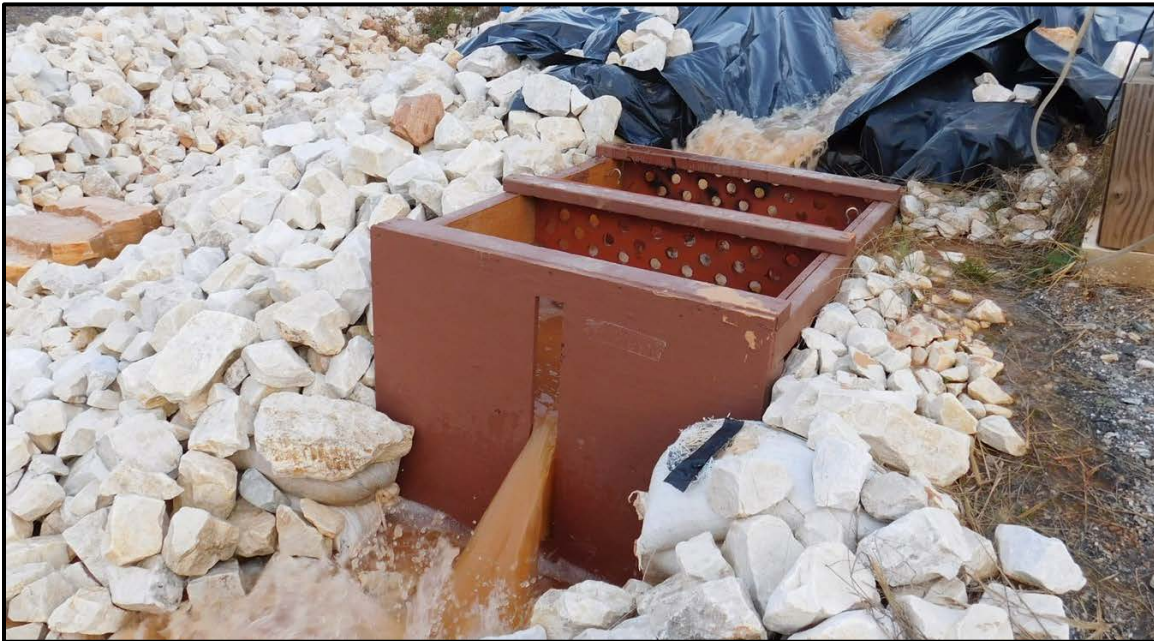
Figure 3.10: Auxiliary Spillway Weir Box.
