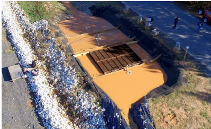
(c) Lamella units installed in the AU-ESCTF sediment basin.
