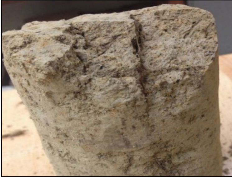
Figure 4.3 Cracks and fissures inside the Shelby tube (IS-2.5) from shallow depth (I-180 and Superior St.)
