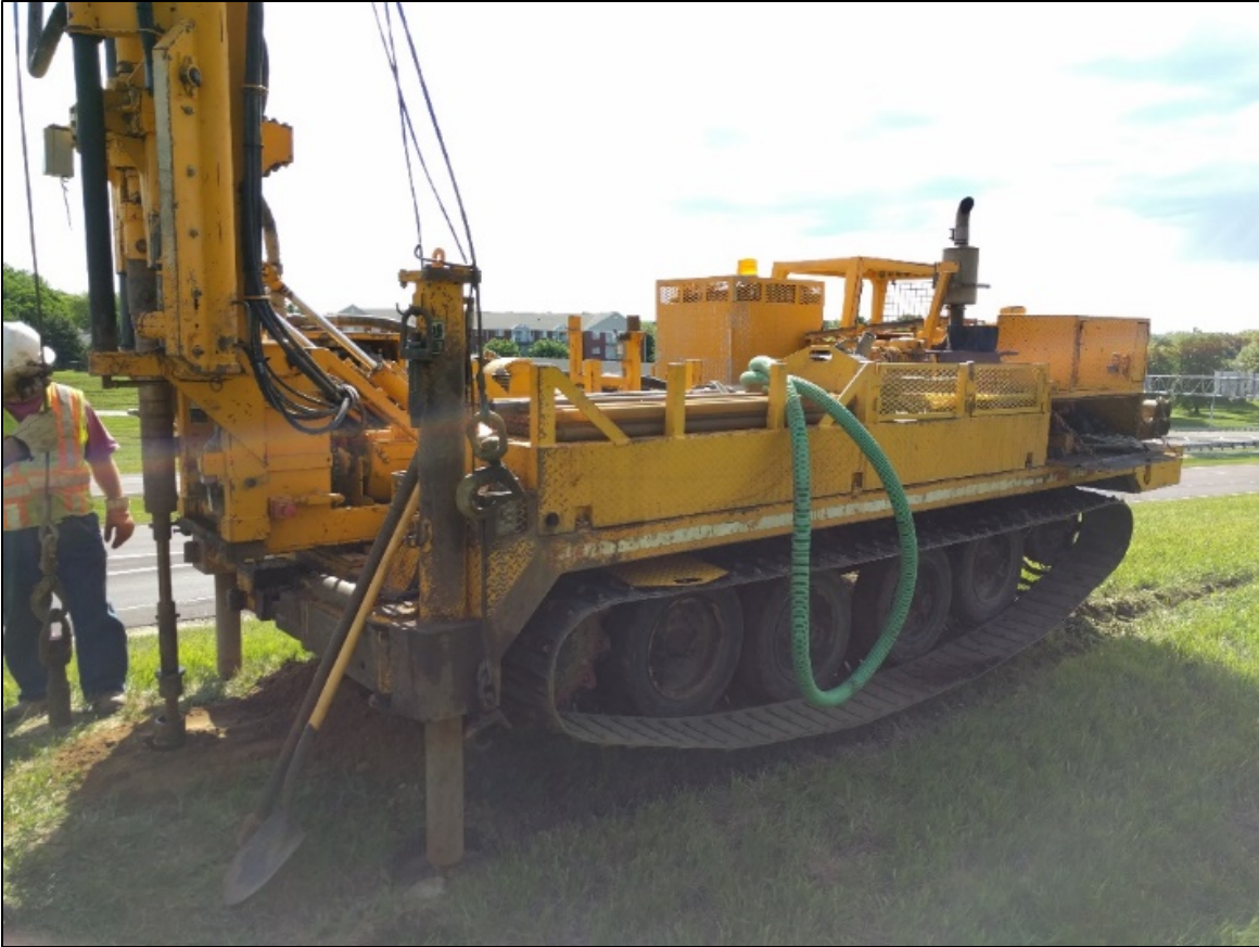
Figure 4.2 Drilling equipment (I-180 and Superior St.)
