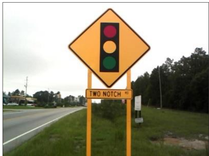
Advance Signal Ahead warning sign with cross street name. Source: SCDOT.
