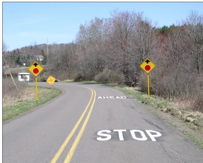
Signage and pavement marking upgrades. Source: PennDOT.
