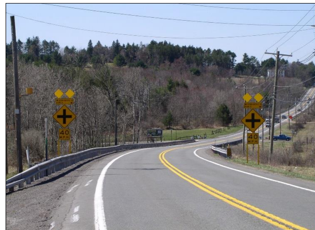
Signage upgrades include doubling up the intersection warning signs, adding cross street names, and yellow flags above the signs. Source: PennDOT.
