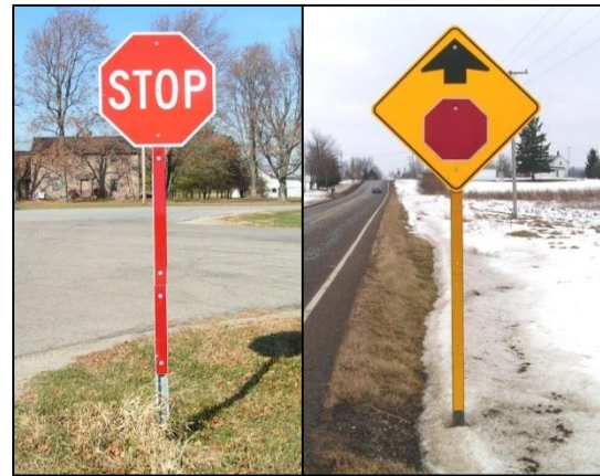
Sign post reflectors were one of the systemic countermeasures that the ISIP identified. Source: ODOT.
