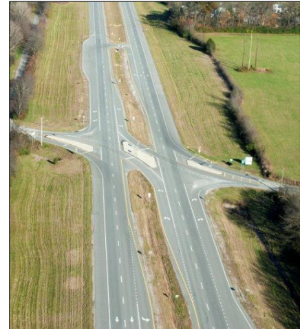
J-Turn Intersection. Source: Tennessee DOT.
