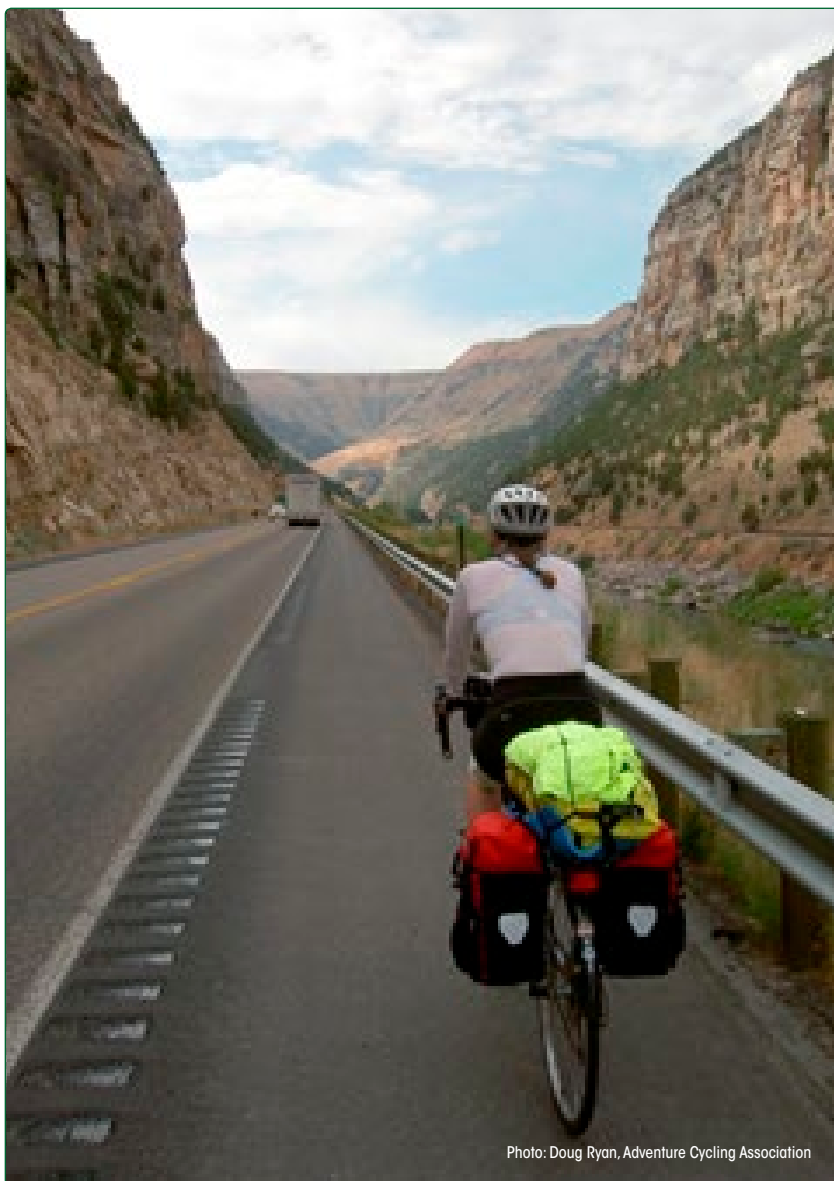
FIGURE 4. Example of Bicycle Gap.
