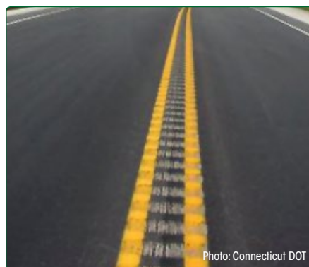
FIGURE 2. Center Line Rumble Stripes.
