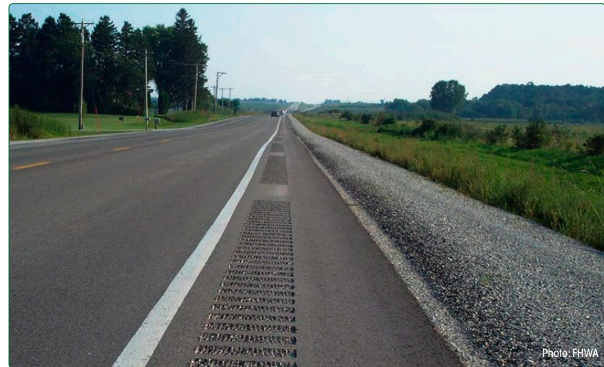
FIGURE 3. Early Shoulder Rumble Strip Installation.
