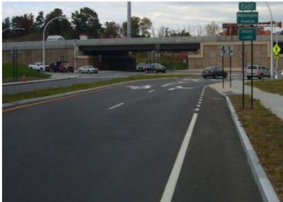
Figure 30. Photo. Street-level view of southern approach on Fuller Rd., Albany, NY.
