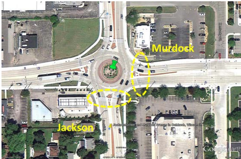
Figure 24. Photo. Aerial view of Jackson St. and Murdock Ave., Oshkosh, WI.
