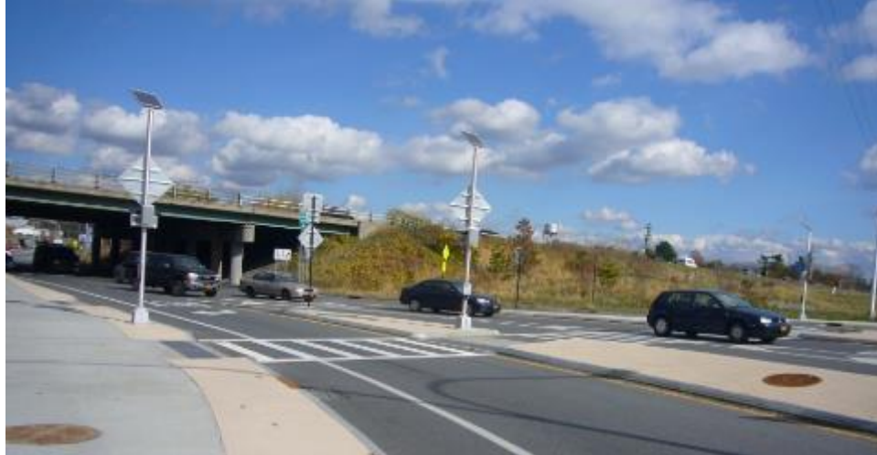
Figure 31. Photo. Street-level view of channelized turn lane on northern approach on Fuller Rd., Albany, NY.
