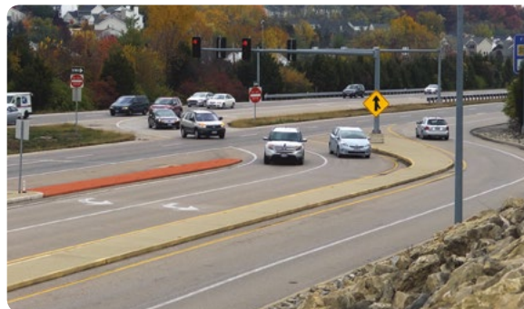
Left Turn Crossover at MO 13 and Summit Drive Source: DLT Case Study Video FHWA-SA-14-055
