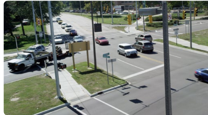
Intersection of Michigan Avenue and South Harrison Road Source: MUT Case Study Video FHWA-SA-14-049
