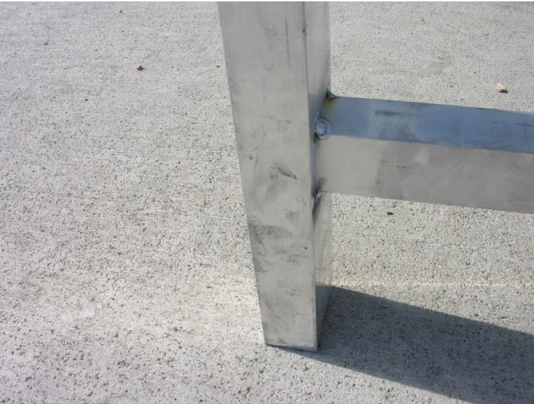
Figure 48. Welded Aluminum Rail, Design Concept AW2
