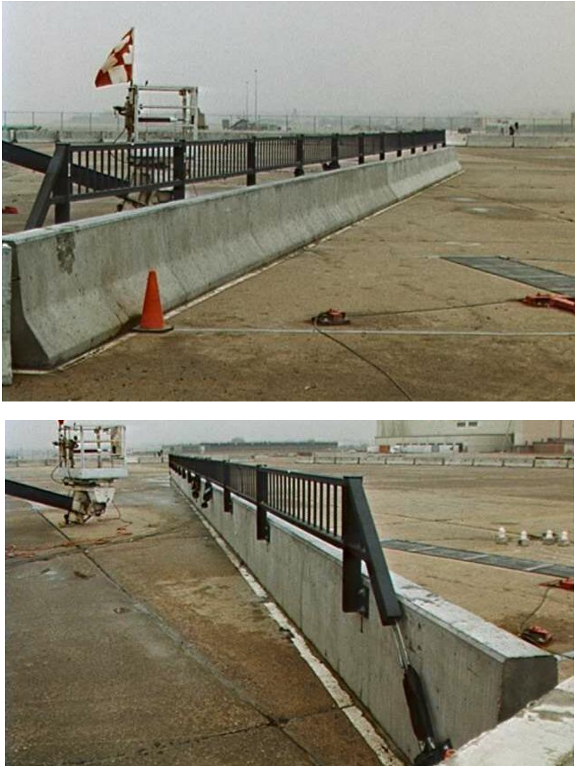
Figure 6. Minnesota Combination Traffic and Pedestrian Barrier [10]
