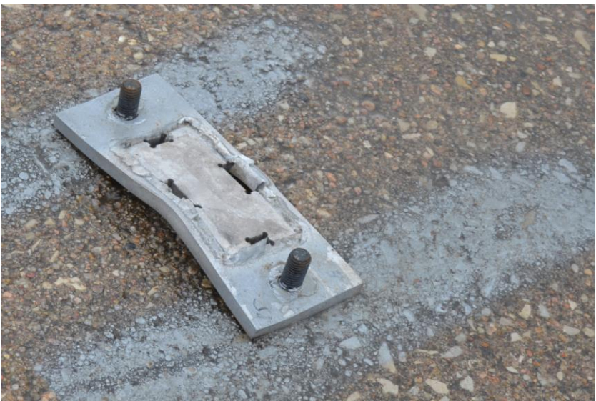
Figure 197. Panel No. 1 Damage, Test No. APR-2
