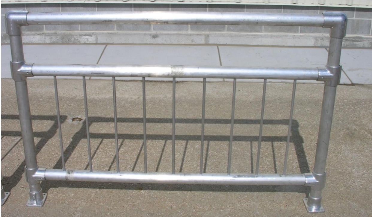
Figure 124. Pedestrian Rail AM-1
