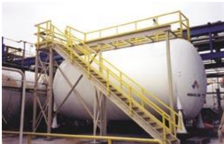
Figure 8. Examples of Existing FRP Handrail Systems [15-17]
