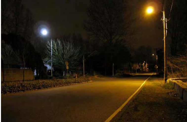
Figure 8. Visual comparison between LED and HPS luminaires at entrance to Lija Loop (Kinzezy and Myer 2009b).
