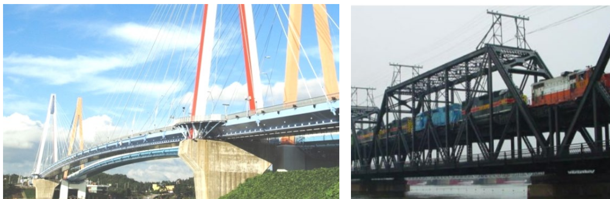
Figure 1.2 Bridges monitored by researchers: (a) Jindo Bridge, (b) Government Bridge
