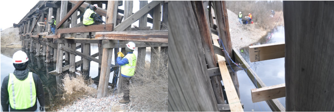
Figure 6.2 Platform built to mount equipment
