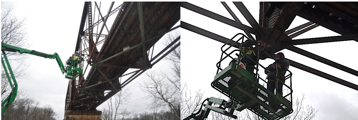
Figure 6.13 Mounting of equipment
