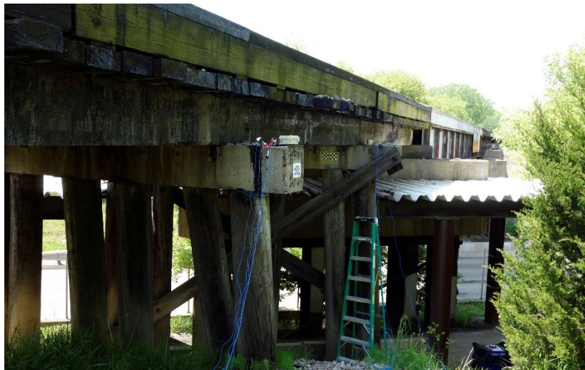
Figure 6.20 Timber trestle bridge setup
