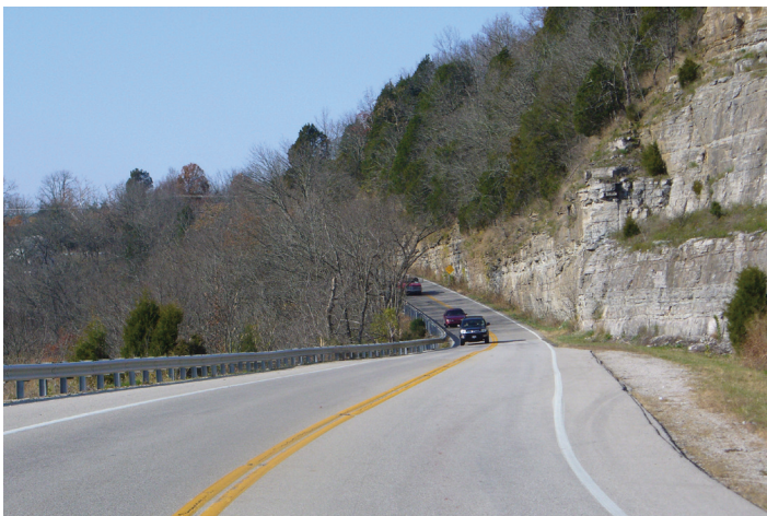
Kentucky's roadways include horizontal and vertical curves and varying shoulder widths.
