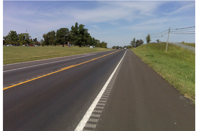
KYTC is installing hundreds of miles of rumble strips/stripes in conjunction with its pavement resurfacing program.
