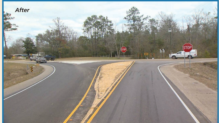
Louisiana installed two oversized STOP signs, a low-cost countermeasure, at this stop-controlled, three-legged rural intersection. Photo: LA DOTD.
