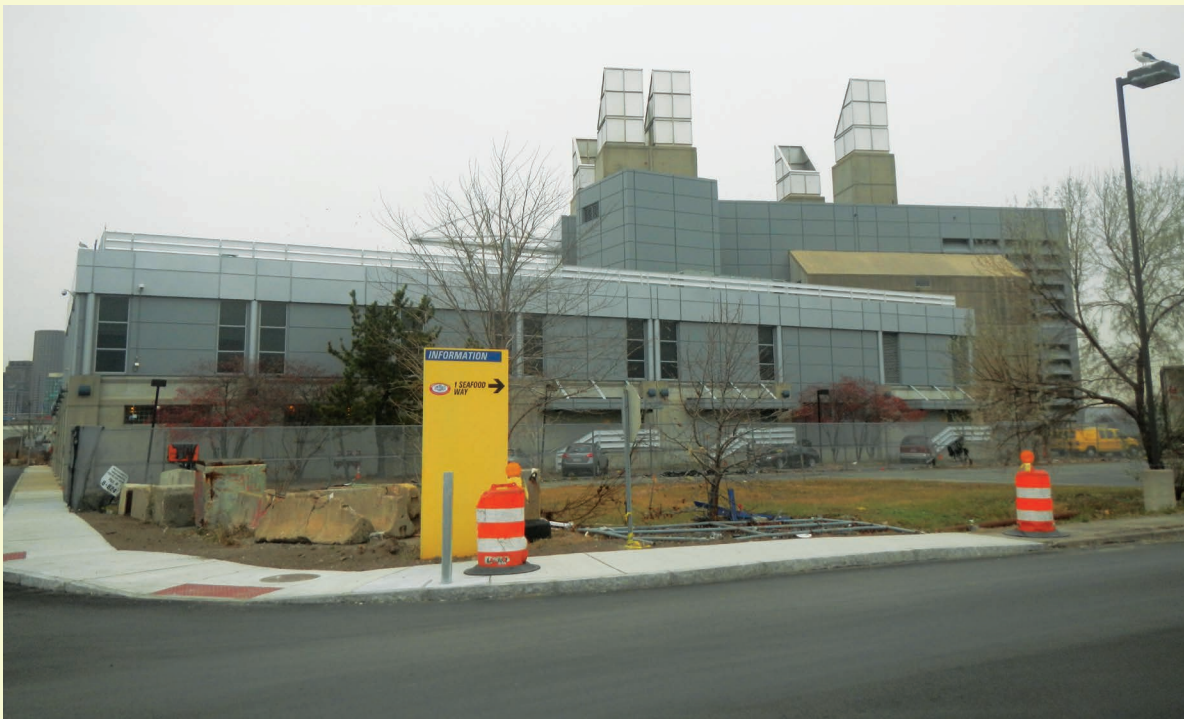
This large vent building for the Ted Williams Tunnel could be vulnerable to flooding. MassDOT has identified local adaptation options to protect this asset from future flooding. Photo: MassDOT.
