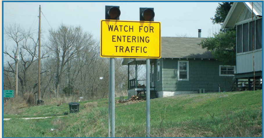
MoDOT installed this “Watch for Entering Traffic” sign on a suburban street near Tunas, MO. Vehicles activate the sign’s flashing beacons by driving over loops in the roadway. This installation is an example of a low-cost safety measure. Photo: MoDOT.
