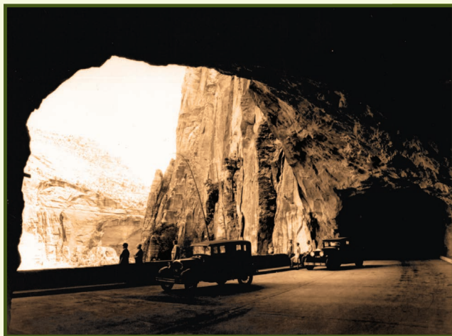
NPS describes the Zion-Mt. Carmel Highway as a "road designed to go where no road had gone before." This historic photograph shows the view looking east from Gallery #2. Photo: AASHTO.
