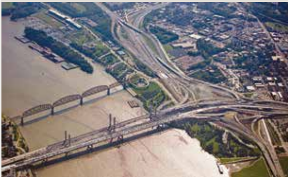
Substantially completed in December 2016, the Ohio River Bridges Downtown Crossing in Louisville, KY, shown here, was financed using GARVEE bonds, toll revenue bonds, and a USDOT TIFIA loan. Photo: Ohio River Bridges Downtown Crossing.
