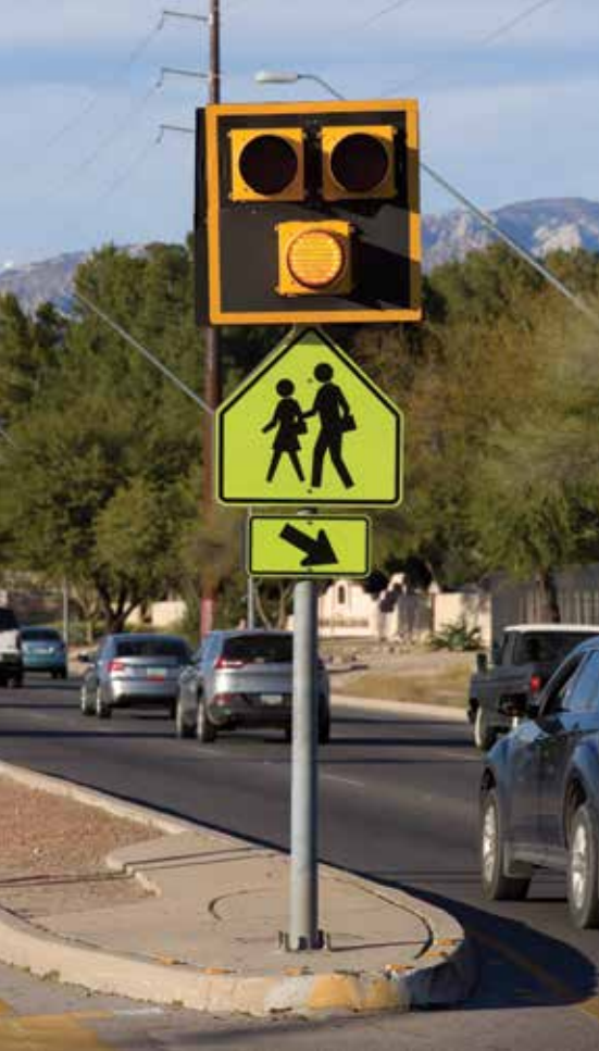
The lower indication on this PHB shows steady yellow, which comes after it shows flashing yellow, alerting drivers to the upcoming need to stop for pedestrians. Photo: Martha Lochert Photography.
