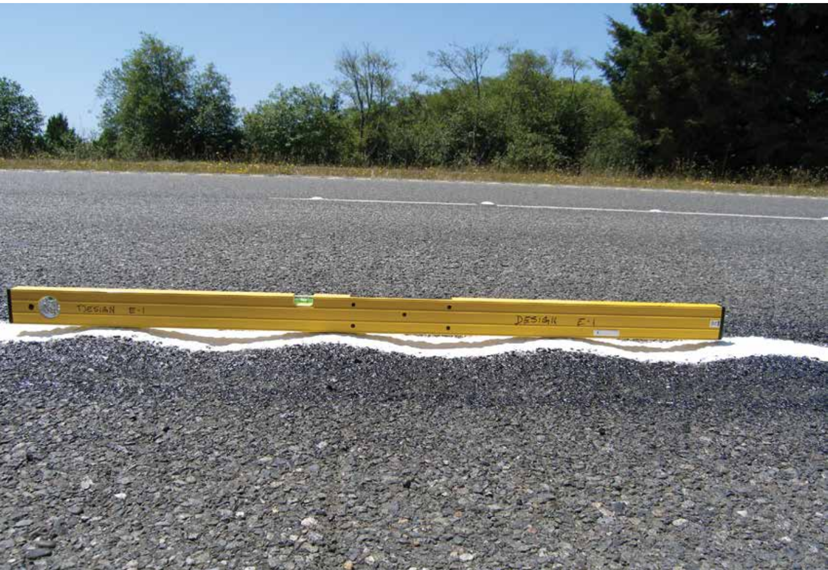
This side view with a long straightedge laid on top of the pavement shows the sinusoidal shape of California's mumble strip design. Photo: Caltrans, Caltrans 2014 Excellence in Transportation Award Winners, Transportation Innovations Category, "Mumble Strip Installation and Evaluation."
