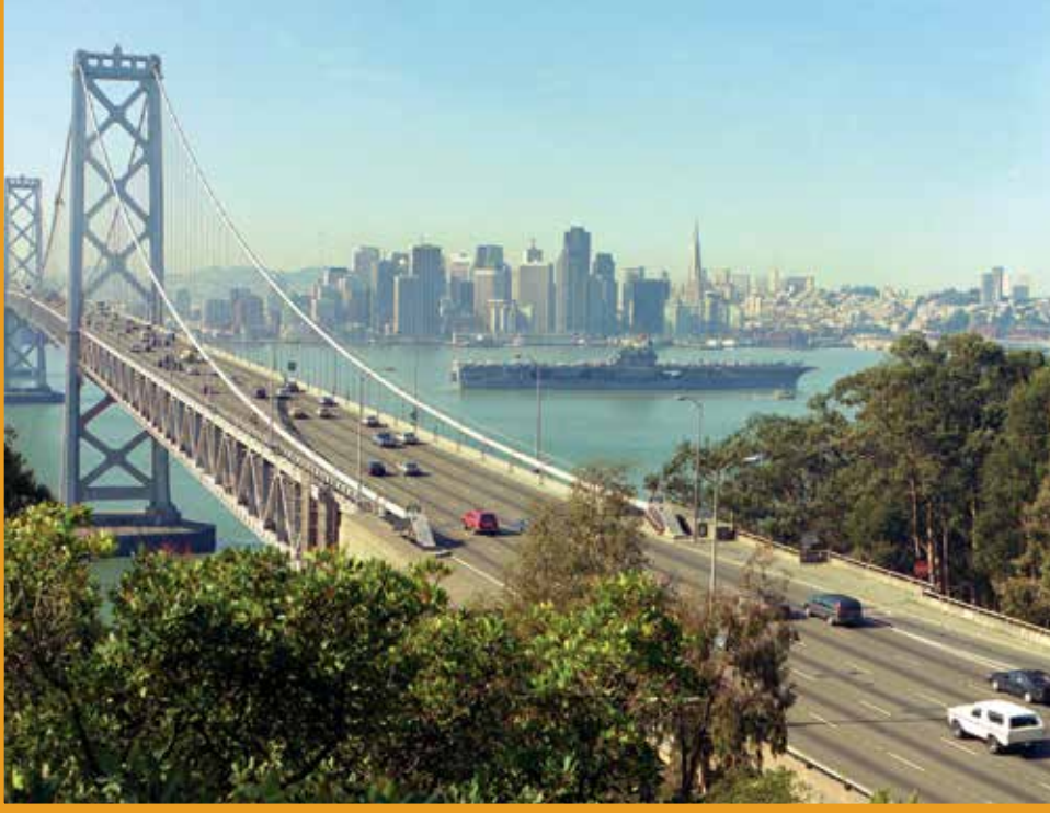
Nearly half of the U.S. population lives in suburban neighborhoods. Metropolitan areas are growing, increasing the need for transportation between cities and their suburbs. Shown here is the Oakland Bay Bridge, which links San Francisco and Oakland, CA. Photo: Department of Defense in National Archives.
