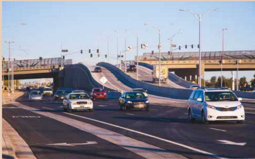
Vehicles travel through the completed interchange project at Bell Road and Grand Avenue (U.S. 60) in Surprise, AZ. This project benefitted from a SHRP2 R09 demonstration workshop. Photo: ADOT.
