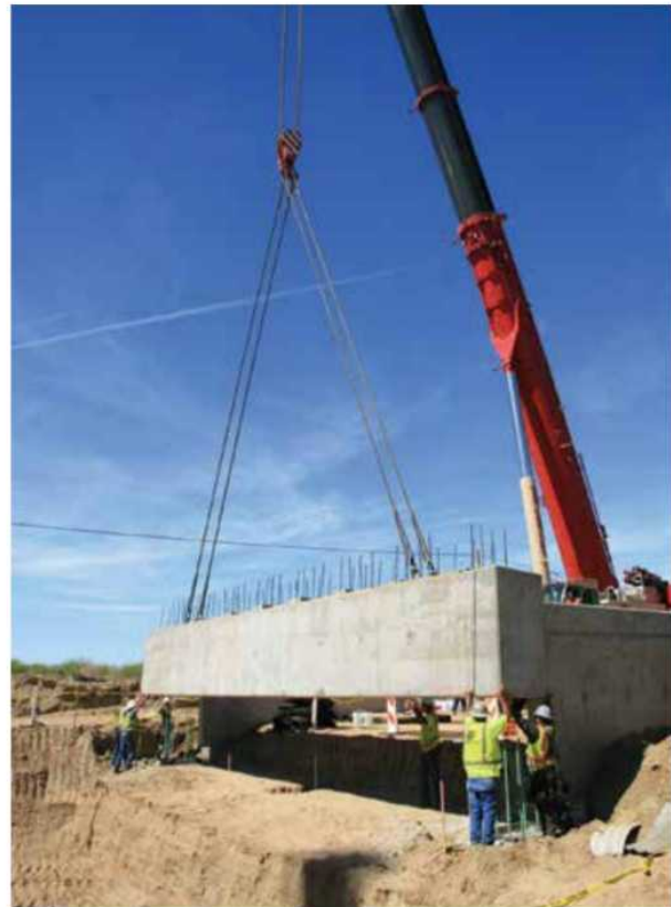
Workers lower a section of Arizona's first prefabricated bridge into place over the Sacramento Wash near Topock, AZ.
