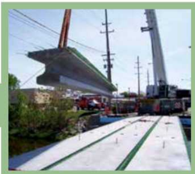
This photo shows the placement of deck bulb-tee girders. Photo: NYSDOT.
