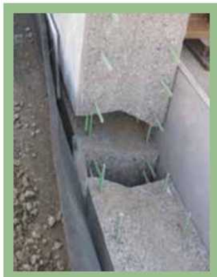
These precast abutment elements will be connected using UHPC. Photo: NYSDOT.
