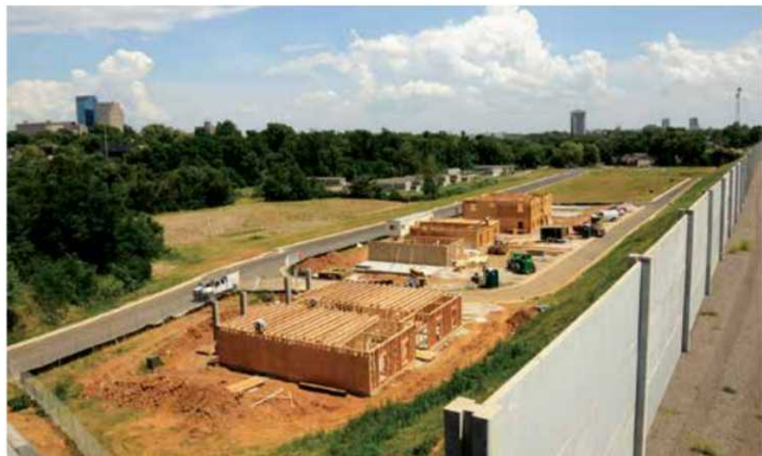
The Newtown Pike Extension in Kentucky involved construction of affordable housing and noise barriers, as shown here, to reduce the impacts on surrounding minority and low-income residential areas.
