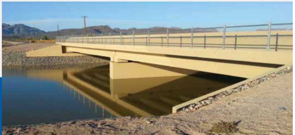
Replacement of the Sacaton Road Bridge, shown here, was procured through a CM/GC contract by the Gila River Indian Community in Arizona. Photo: Gila River Indian Community.
