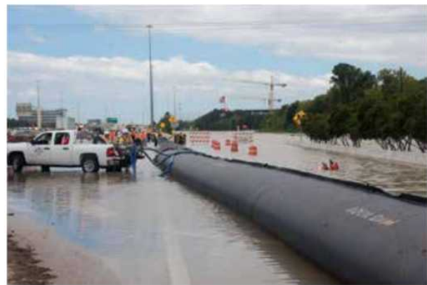
Crews install an AquaDam barrier on flooded Texas roads after Hurricane Harvey in summer 2017.
