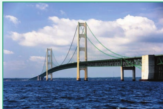
Prototypes of the PFG sensor and protective box were deployed on the Mackinac Bridge, shown here. Engineers and the university research teams installed the sensors on the cross beams in the main suspended span. Photo: Mackinac Bridge Authority.
