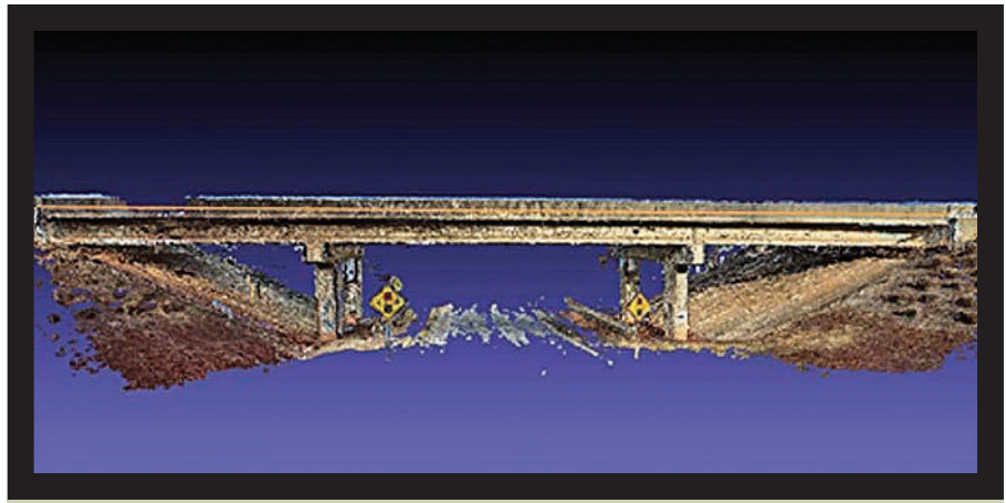
This image of a bridge is created via photogrammetry to permit 3D analysis of the structure for virtual bridge inspection. Photo: Ruodan Lu, Ioannis Brilakis, Campbell Middleton.
