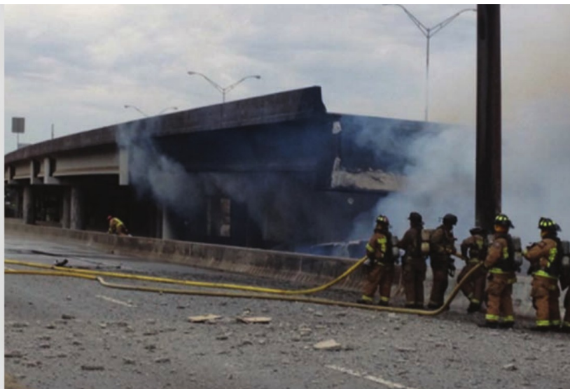
As emergency responders extinguished the flames, GDOT's contractor was already working to provide signage and barricades for traffic control. © GDOT.
