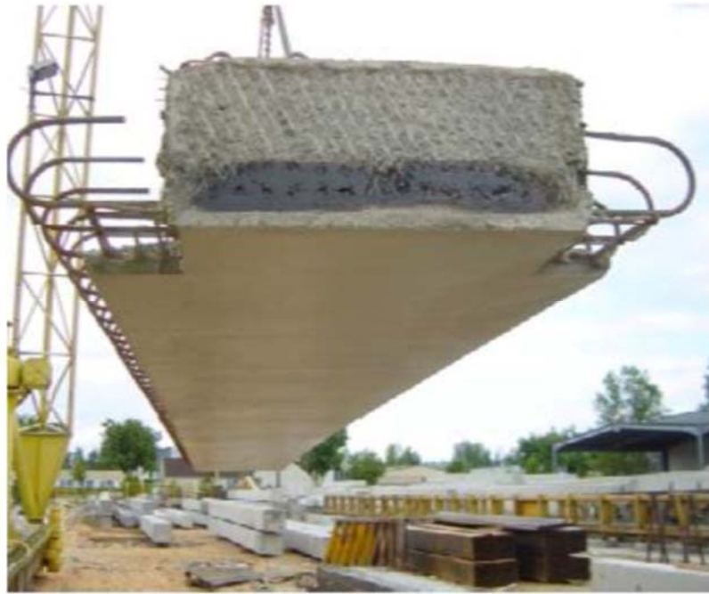
Figure 1-1: Poutre-Dalle system (Bell, 2006)
