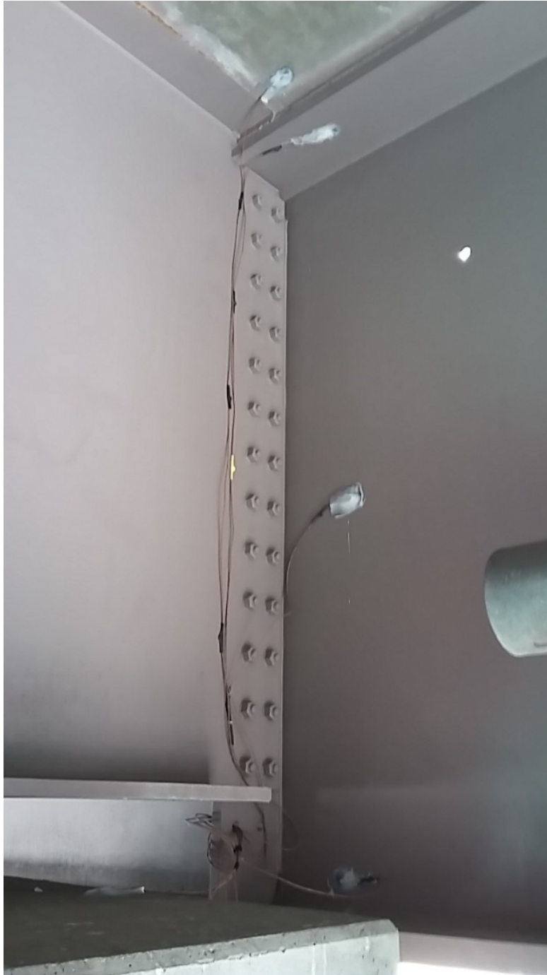
Figure 3.11 Thermocouples that are attached to the girder and to the concrete with epoxy
