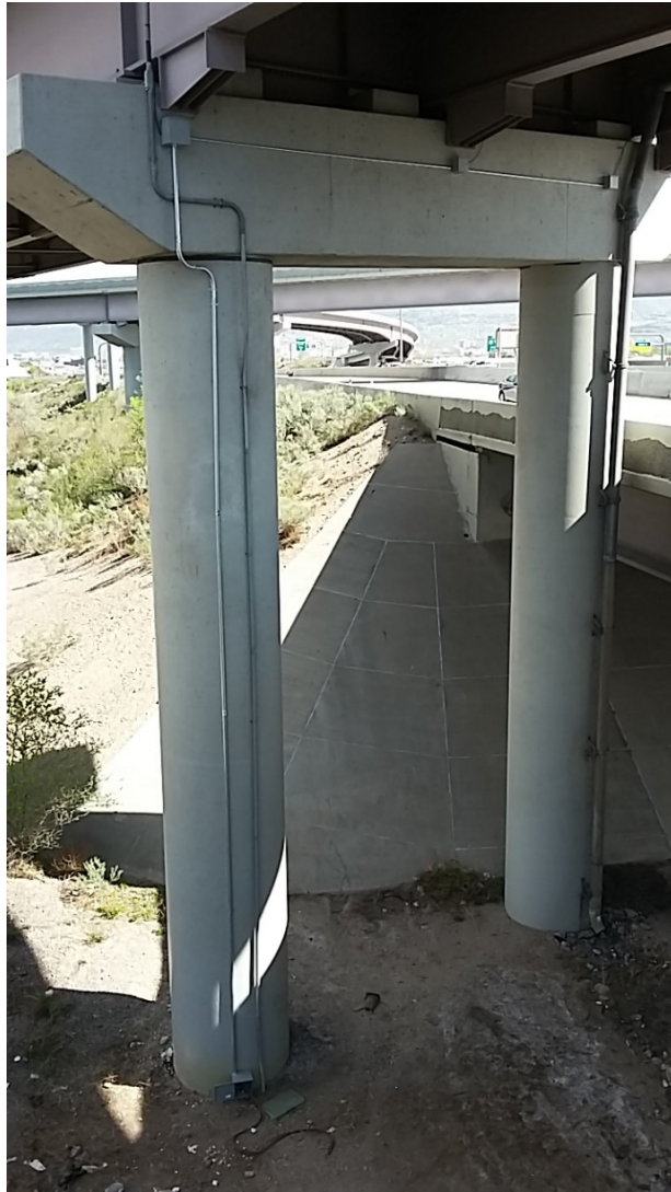
Figure 3.7 Bent number 9, and its columns
