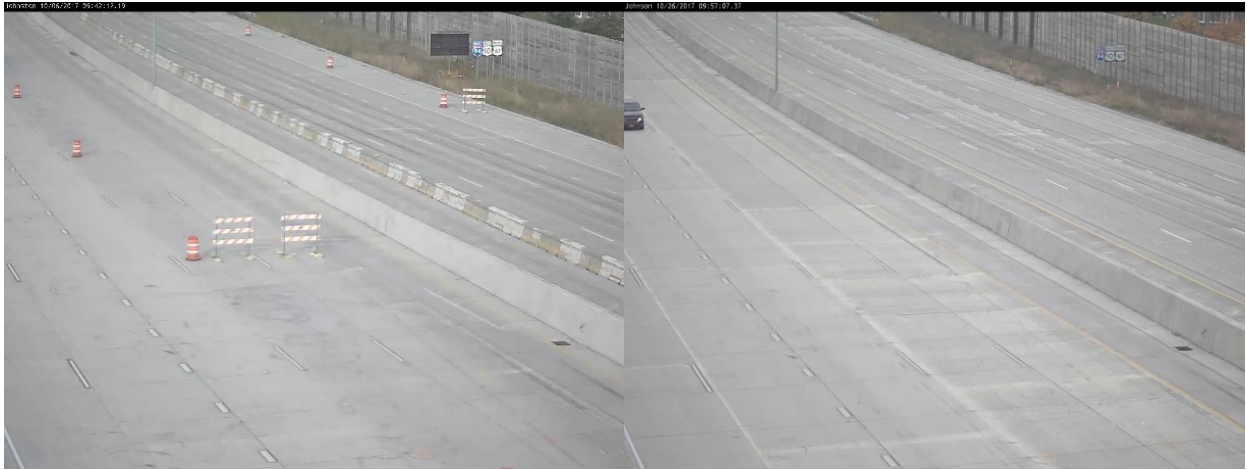
Figure 5.2 Johnson Pkwy Station. All Lanes Open Layouts. 4-Lanes No Shoulder, Normal Road
