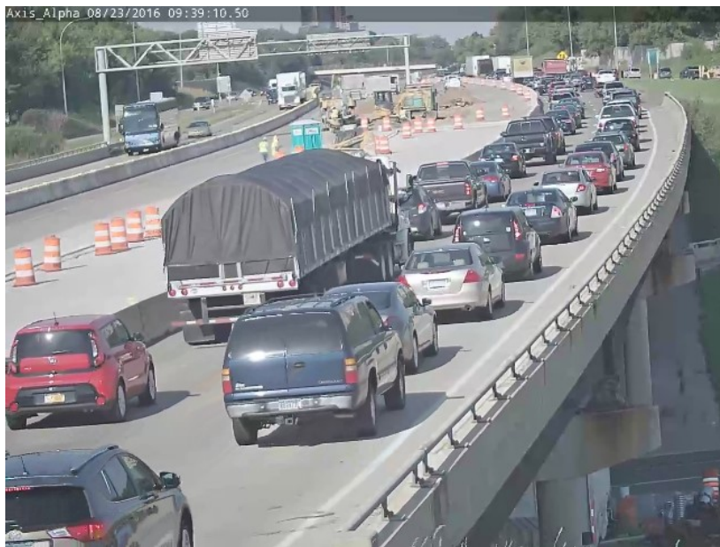
Figure 3.9 Conditions on TH-61 while VMS displayed "Stop Traffic Ahead"
