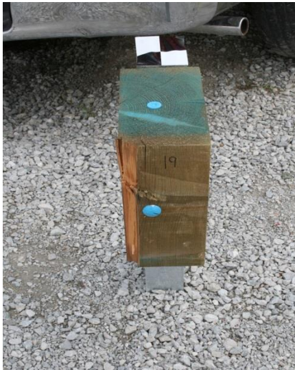
Figure 76. Damage to Post Nos. 17 through 19, Test No. MGSLS-2
