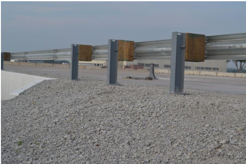
Figure 38. Test Installation, Test No. MGSLs-2
