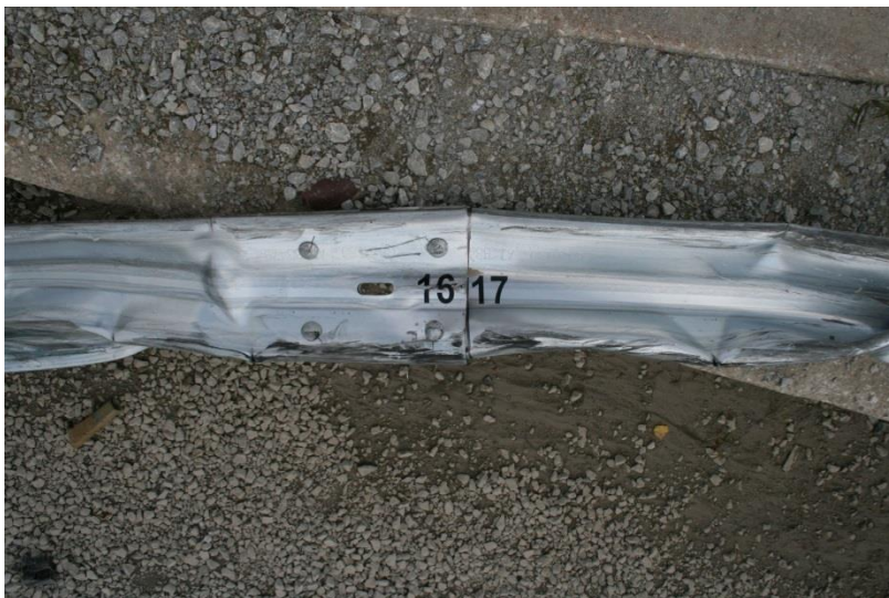
Figure 75. Damage at Post No. 16 and Splice 16-17, Test No. MGSLS-2
