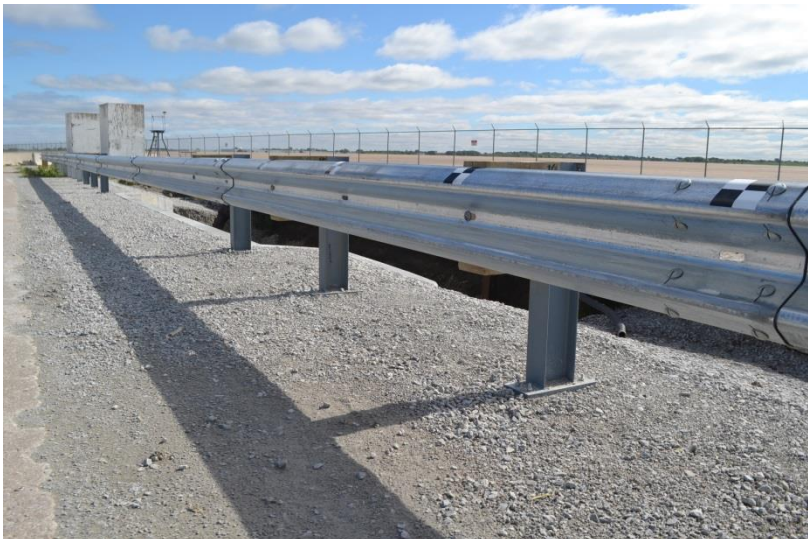
Figure 34. Test Installation, Test No. MGSLS-1
