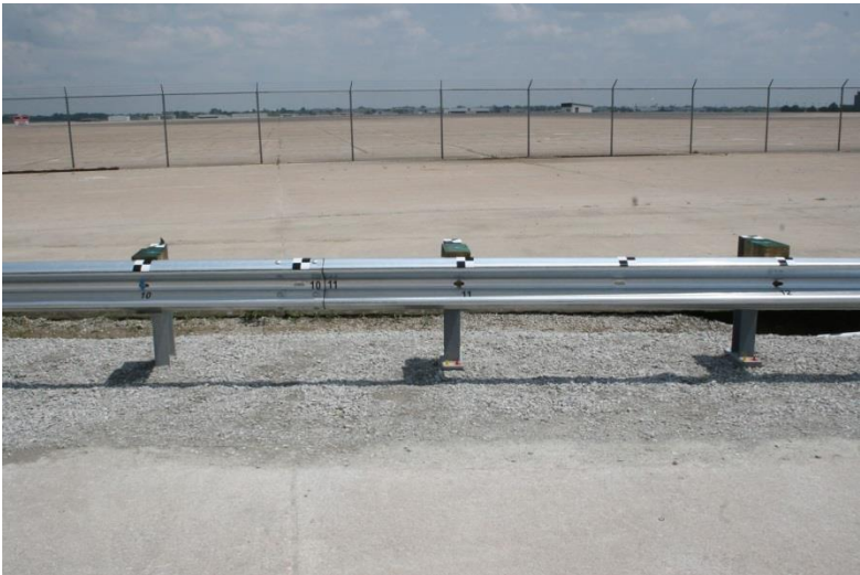
Figure 70. System Damage Between Post Nos. 3 and 12, Test No. MGSLs-2
