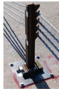
Figure 36. Slip Base Post Assembly and Finite Model
