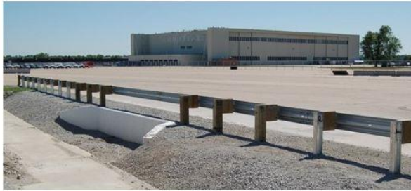
Figure 1. Midwest Guardrail System 25-ft Long-Span Design
