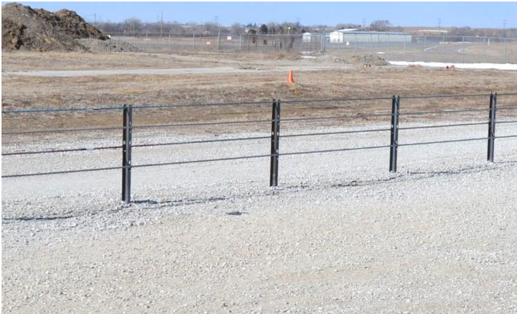
Figure 1. Current Cable Median Barrier Prototype
