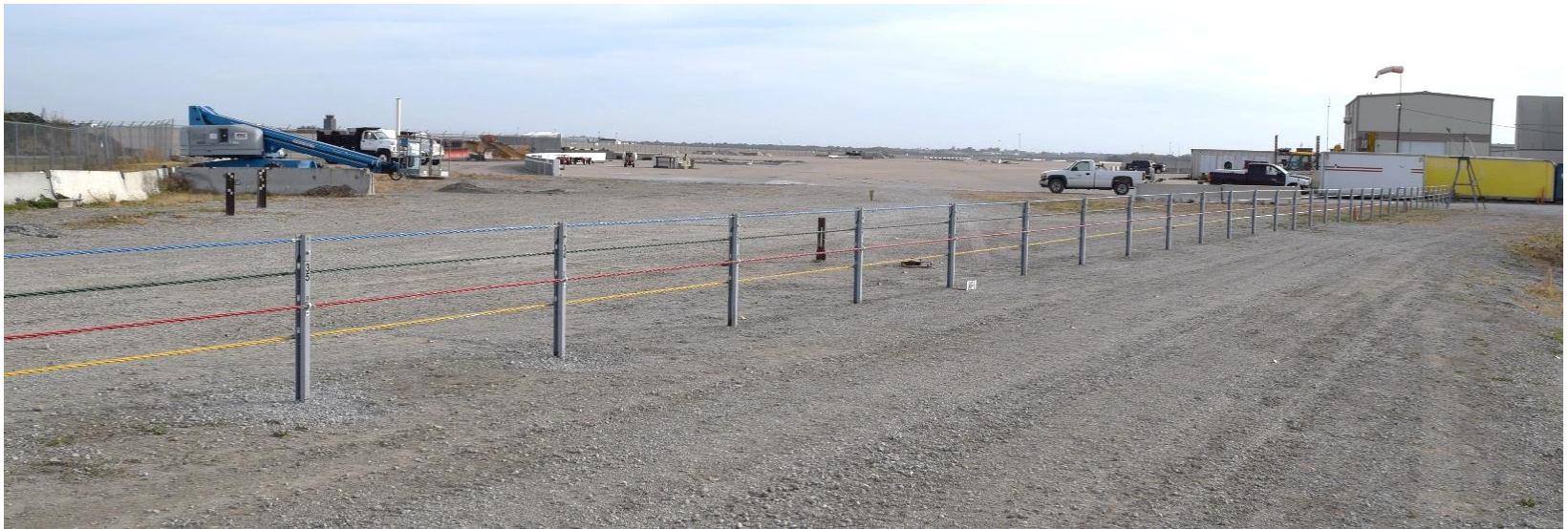
Figure 27. System Installation, Test No. MWP-9
