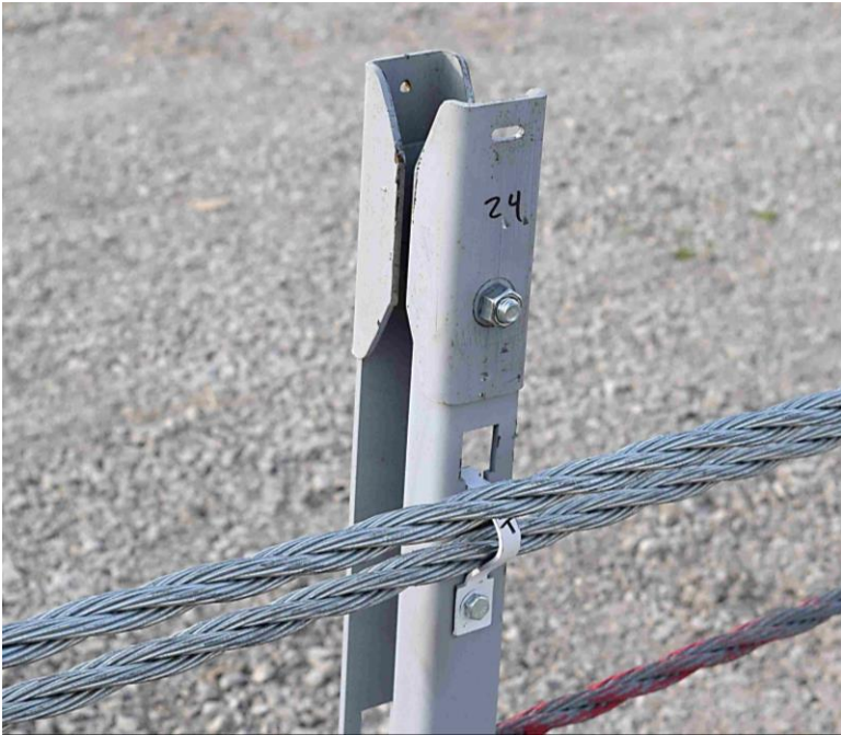
Figure 56. Post No. 24 Damage, Test No. MWP-9
