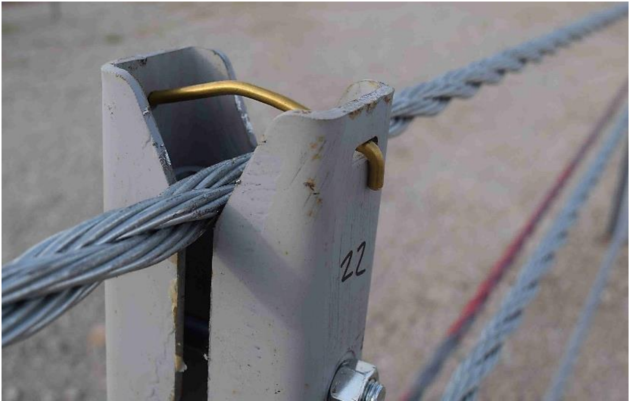
Figure 54. Post No. 22 Damage, Test No. MWP-9
