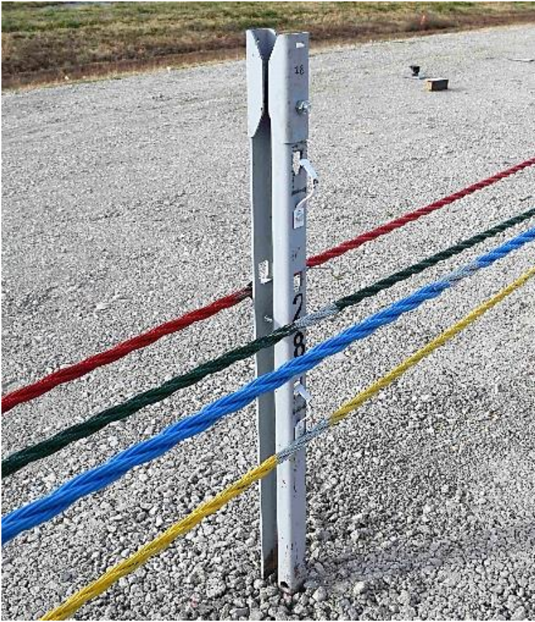
Figure 60. Post No. 28 Damage, Test No. MWP-9
