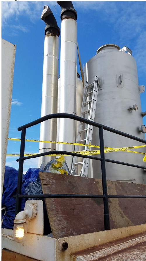
Scrubber before stack reinstalled
