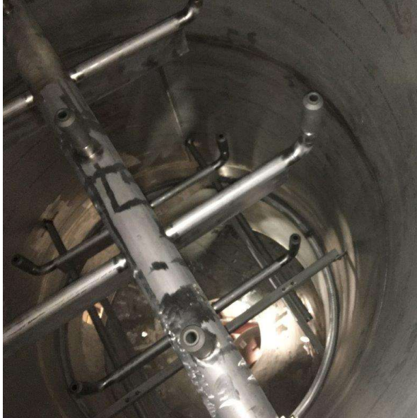
A view into the Scrubber vessel during fabrication
