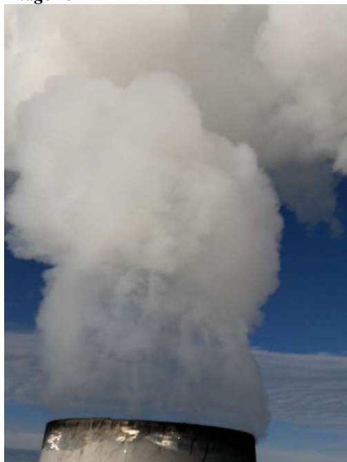
Scrubbed exhaust – a plume of steam
