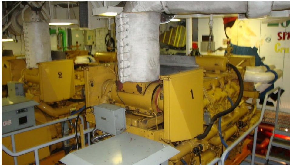
Figure 4. T/S STATE OF MICHIGAN engine room
