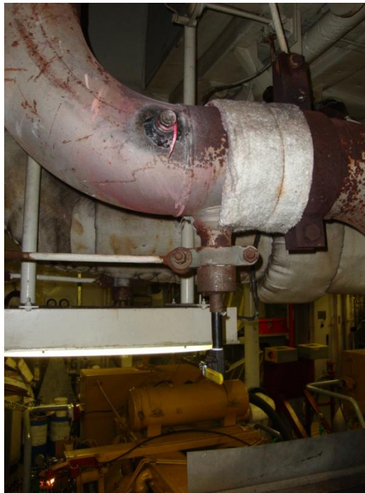
Figure 11. Exhaust Trunk Modification
