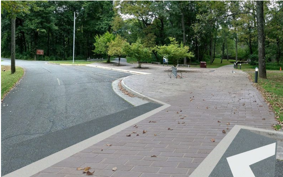
Figure 3-11: Traffic Calming Location 5 – photo rendering (Note: two raised crossings, one in the in foreground and one in the background) Source: Volpe
