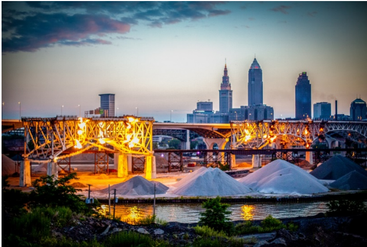
Figure 3: The steel skeleton of the old Innerbelt Bridge was demolished using explosives in July 2014. In total, 19,775 tons of steel and steel rebar were recycled from the old bridge. (Image courtesy of Marianne Mangan)
