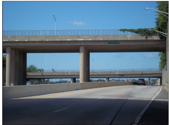
Figure 1: Fulton Avenue Bridge spans the "highway to nowhere" and connects bisected West Baltimore neighborhood (Image courtesy of FHWA).
