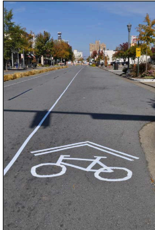
Figure 2: In the full-size mockup, hay bales (upper left) provided a visual suggestion of what a median might look like. Duct tape delineated temporary bicycle lanes.
