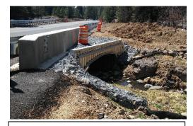
A bottomless culvert was installed under NM-434 to connect Big Blue Creek, a tributary to Coyote Creek, with NM-434. Source: FHWA
