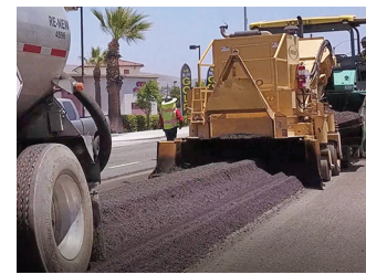
Pavement Recycling Systems Figure 4. Cold in-place recycling
