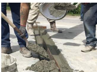
ACPA Figure 9. Partial-depth repair
