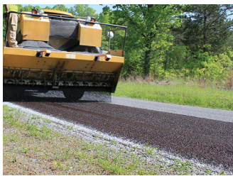
Slurry Pavers, Inc. Figure 1. Chip sealing
