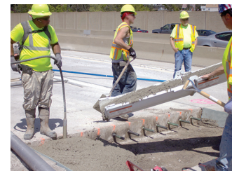
ACPA Figure 8. Full-depth repair
