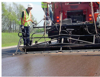
National Center for Pavement Preservation Figure 2. Micro surfacing
