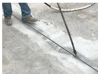
Dow Corning Figure 11. Joint sealing
