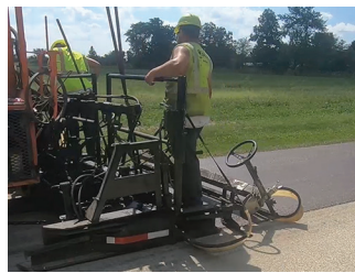
Strawser Construction Inc. Figure 3. Cape sealing
