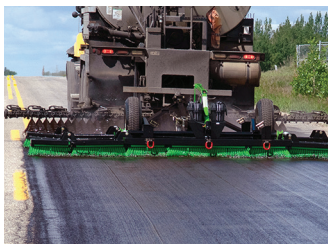
Saskatchewan Ministry of Highways and Infrastructure Figure 5. Scrub sealing
