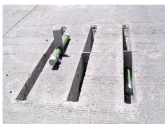
ACPA Figure 10. Dowel bar retrofit
