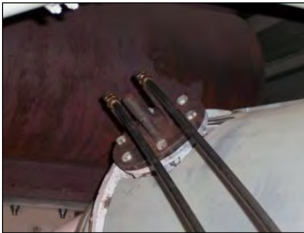
(b) Exhaust sampling port
