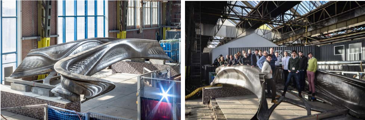
Figure 17 MX3D 3D printed constructed a steel bridge (Block 2018).
